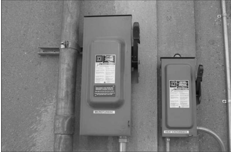
*Typical 480 v manual disconnect with a visible open*
