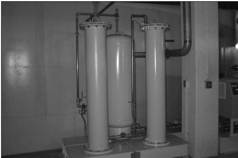
*Typical biogas siloxane removal system*
