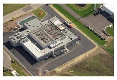
and then supplied to two gas engine generators that generate 3.2 MW of electricity that is sold to Xcel Energy for distribution on their grid. The heat is captured from the engines and transferred back to the adjacent food processing facility.
